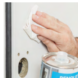
3. Cleaning and smoothing
